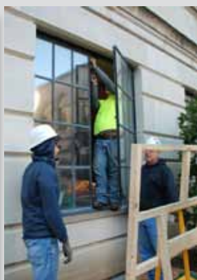
Above, contractors remove windows from first and second floors for repair and repainting.
