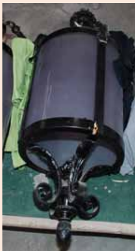
Above, left, a corridor light with the black paint applied sometime prior to 1970, and right, the corridor light after cleaning. The original bronze finish will be waxed to highlight and protect the fixture surface.
