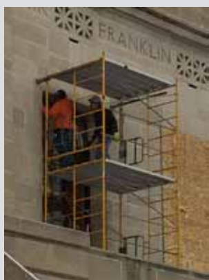
Above, contractors remove windows from first and second floors for repair and repainting.
