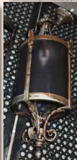
Above, left, a corridor light with the black paint applied sometime prior to 1970, and right, the corridor light after cleaning. The original bronze finish will be waxed to highlight and protect the fixture surface.
