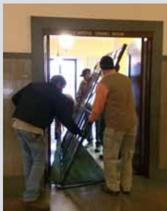
Above, a repaired and repainted test window is returned and, at right reinstalled. Above right, the steel jambs are precisely installed so that all hinge hardware is in alignment and the latch hardware fits properly. The securely closed latches will hold tight and help minimize air loss.
