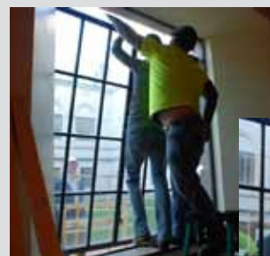
Above, first floor window removal goes smoothly. Right and below right, contractors easily set the window out and onto a cart to take it to the truck which will move the securely strapped windows to the repair shop.
