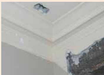
Above, crown molding in the south center corridor was hidden by dropped ceiling for years. Right, a removed section of the molding allows staff to conduct paint analysis and plan for repair and restoration of this detail.
