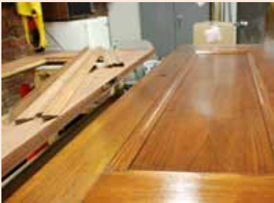
Above, two doors in the finish shop. Disassembled pieces are kept together during the refishing process. Then the doors and trim are labeled with room numbers and stored, right, to await reinstallation after each phase of the project is completed.
