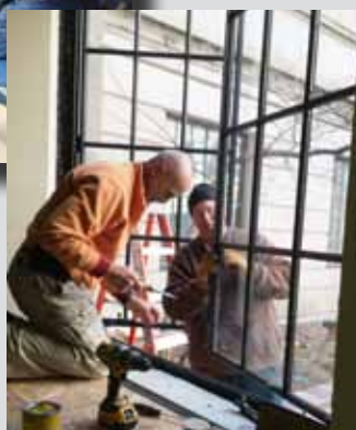
Above, a repaired and repainted test window is returned and, at right reinstalled. Above right, the steel jambs are precisely installed so that all hinge hardware is in alignment and the latch hardware fits properly. The securely closed latches will hold tight and help minimize air loss.
