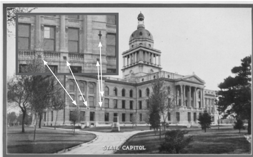
The arrows in this image of the second Capitol, and inset, show the makeshift tension washers installed to hold the building together as it began to settle and structurally fail. The Legislature would soon propose to build a third Capitol.
