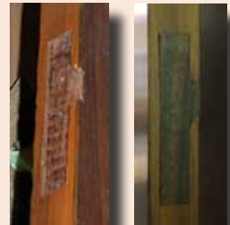
Above left, after carpentry staff removed the improperly located door, OCC mason Dan Kratky began work preparing for the reinstallation of the door and restoring the corridor floor to its original condition. Above right, the door and floor restored.
