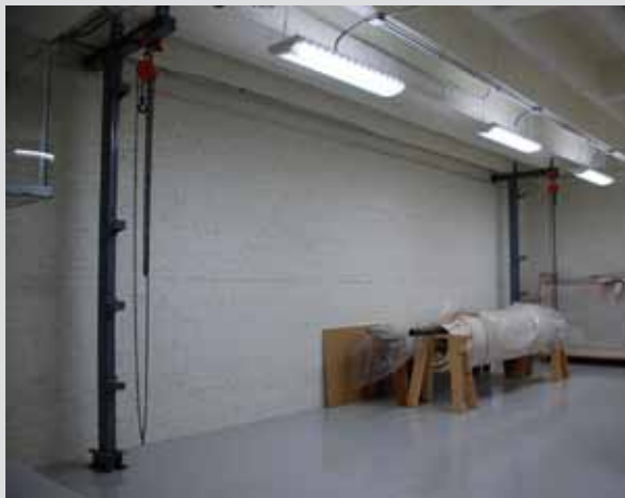
Above, one rug has been placed in temporary storage in the newly completed space. This rug rests on saw horses and a small metal pipe, the previous method of storage, which put stress on the rug. Right, each support frame is bolted to the floor and ceiling for stability. The rugs to be stored may weigh up to 1000 pounds. For ease of placement and access, preservation architects devised a special trolley system to raise and lower the bar joists into place on the brackets.
