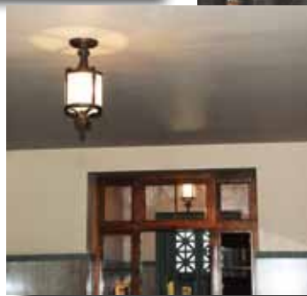
Left, the two restored lamps in the south entrance vestibule and corridor are the first of many to be returned to their original location. The plaster ceiling in this area is original and will be replicated throughout the first floor. Above, once the lay-in ceiling is removed, the lamps will be repaired and restored with the lengthened chains, right, to allow all first floor corridor fixtures to hang at a uniform height.
