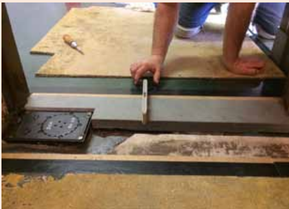
Above, after installing the door closer and adding concrete to hold it in place, fill voids, and level the floor, Kratky sets the slate threshold. The linoleum will be cleaned of glue, foreground, and repaired. Right, OCC keeps a stock of the Battleship Linoleum, some removed from service due to changes in adaptive use space. These pieces are then used to repair damage in other locations where the durable material is still functional.
