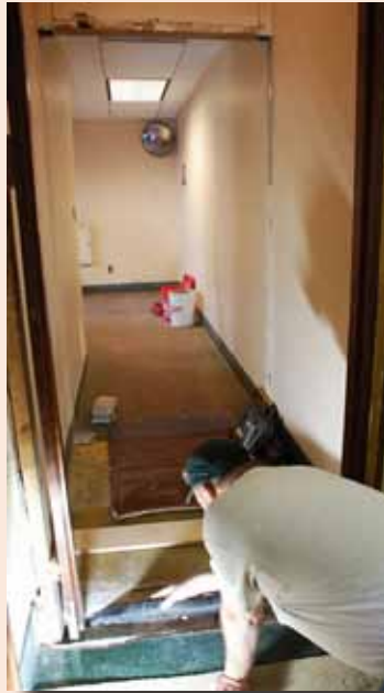
Above left, after carpentry staff removed the improperly located door, OCC mason Dan Kratky began work preparing for the reinstallation of the door and restoring the corridor floor to its original condition. Above right, the door and floor restored.
