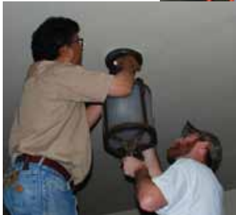
Right, maintenance staff prepare to install a restored lamp in the south center corridor. Below, Tahir Karimi and Zac Hanna work together to secure the lamp using the new decorative acorn cap-nuts patinated to match the restored finish.
