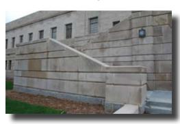
The west promenade stair, newly restored, appears to be constructed of granite and limestone. The concrete and brick core are hidden from view
