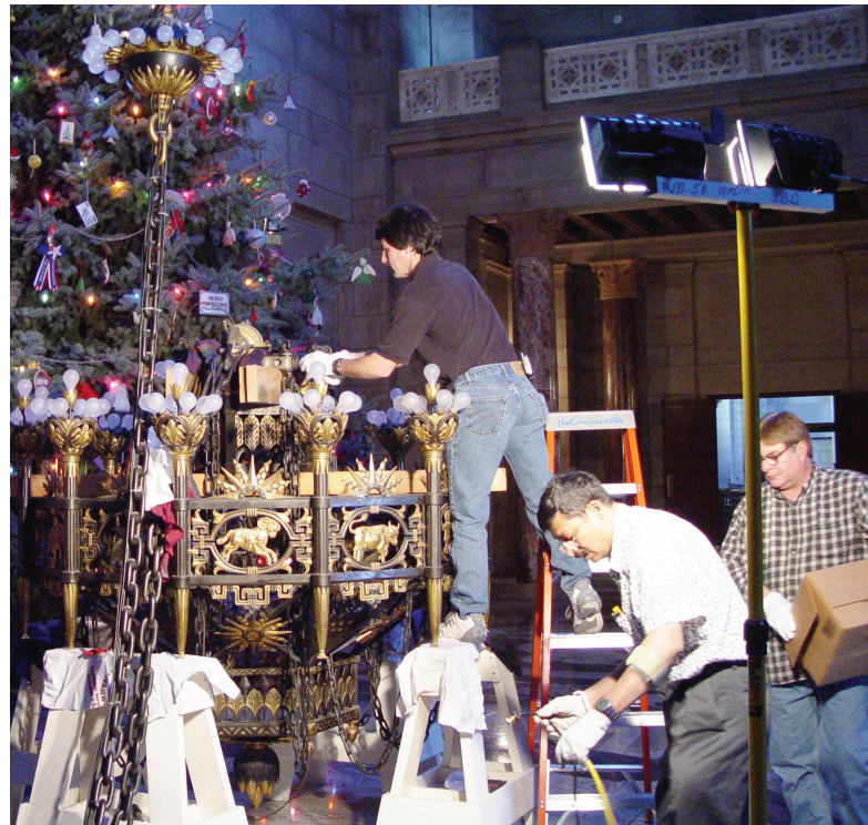
Brett Daugherty, Facility Maintenance Supervisor, climbs above the Rotunda chandelier as John Steele, Facility Maintenance Specialist and Tahir Karimi, Capitol Electrician, help change the 136 light bulbs in the Rotunda's 3,500 pound chandelier. The signs of the zodiac encircle the chandelier and represent the passage of the seasons.
