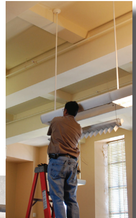
Tahir Karimi installs a new ballast in a tower fluorescent fixture.
