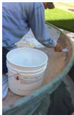
Left, tile designer, Doug Harris at the Bisazza studio in Florida created the pattern in small panels, allowing gaps in the outer edge to accommodate the bowl’s curve. The bowls were stripped to bare bronze to provide maximum adherence. Simulated weather testing revealed the commonly available grouts used for tile were too rigid; expansion and contraction caused the glass tile to crack. Above, a flexible adhesive, similar to that used to hold tiles on the space shuttles is applied to the bowl. Above right, each panel of tile had a brightly colored placement number attached so they could be laid according to the pattern.
