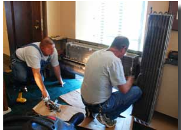
Above, shop staff put the finishing touches on a newly installed induction unit. The unit leaning on the right could not be repaired.
