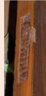
Above, most doors in the Capitol operate with a hydraulic door closer to prevent slamming. During his floor work Kratky uncovered the original door closer location which had been filled with mortar and covered with carpet, and reused the original hole. Above right, changing the location and operation of the door required the addition of hinges. Installing hinges in the original door was very crudely done. Carpentry staff filled in the hole during the restoration of the door.
