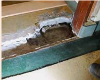
Above, most doors in the Capitol operate with a hydraulic door closer to prevent slamming. During his floor work Kratky uncovered the original door closer location which had been filled with mortar and covered with carpet, and reused the original hole. Above right, changing the location and operation of the door required the addition of hinges. Installing hinges in the original door was very crudely done. Carpentry staff filled in the hole during the restoration of the door.
