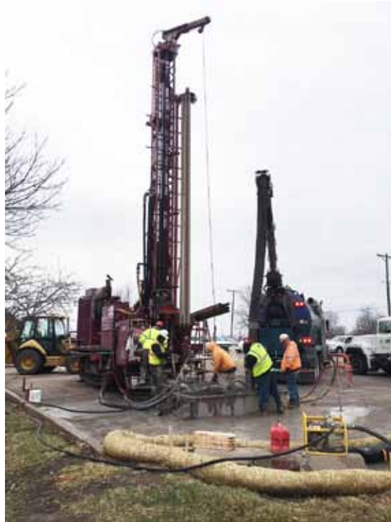
Above: Test wells drilled on the wellfield site in March allowed engineers to study the subsoil structure and plan for the most efficient configuration of the geothermal wells.
