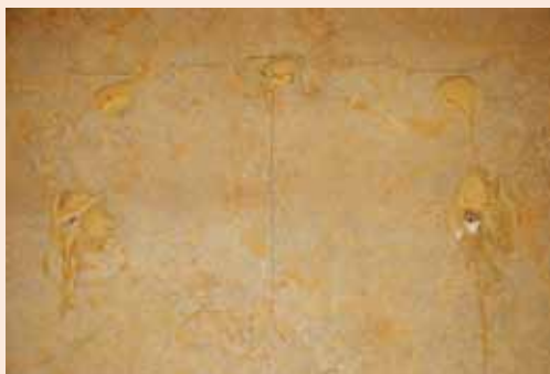
The above left image shows the Kasota stone wall immediately after plaque removal and the liberal application of adhesive. The above right image shows what the wall looked like with adhesive removed prior to complete cleaning.
