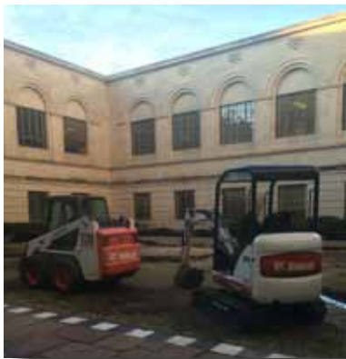
The project so far, above, contractors salvaged original stone pavers, stockpiled them on pallets seen in the upper right of the photo and use a Bobcat equipped with a jack hammer to break up the existing concrete sidewalk base. Left, a small backhoe will be used for excavation in the courtyard.
