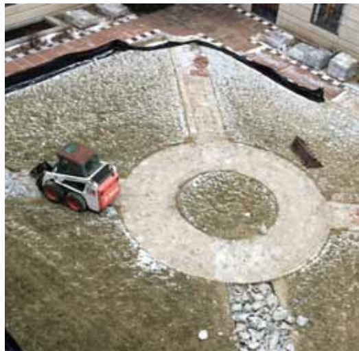
The project so far, above, contractors salvaged original stone pavers, stockpiled them on pallets seen in the upper right of the photo and use a Bobcat equipped with a jack hammer to break up the existing concrete sidewalk base. Left, a small backhoe will be used for excavation in the courtyard.
