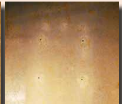
The above left image shows the Kasota stone wall immediately after plaque removal and the liberal application of adhesive. The above right image shows what the wall looked like with adhesive removed prior to complete cleaning.
