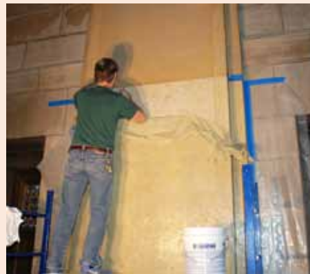
The above left image shows the Kasota stone wall immediately after plaque removal and the liberal application of adhesive. The above right image shows what the wall looked like with adhesive removed prior to complete cleaning.
