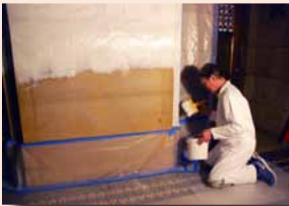
Left, Lagoni applies the latex and detergent poultice to clean a section of the pier where the plaque hung. Right, after drying for forty-eight hours the poultice was peeled away to reveal a very clean piece of stone.
