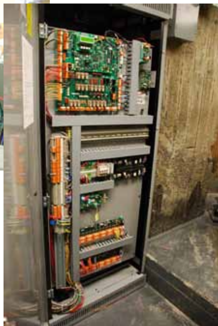
Above, a single computerized control panel has replaced two large mechanical switch panels, left, to control elevator movement.
