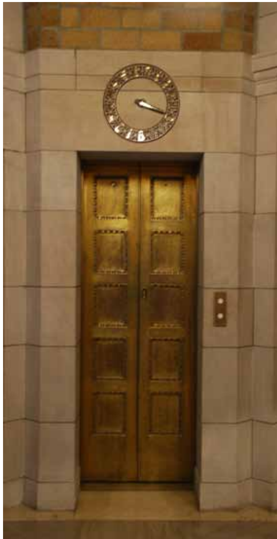
The third floor southwest elevator vestibule with dial installed.
