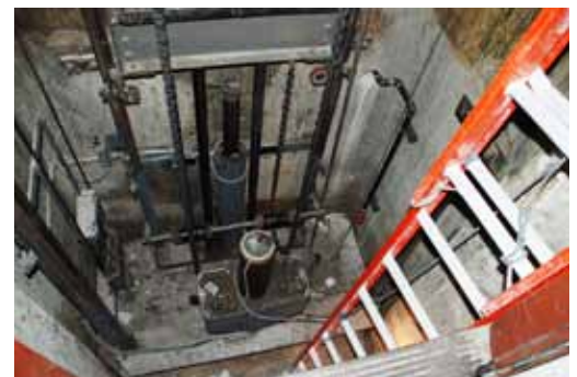
Looking into the elevator shaft at basement level reveals the new buffers, below, which would slow and stop the elevator in a fall. Above, the elevator shaft open to the 14th floor level.
