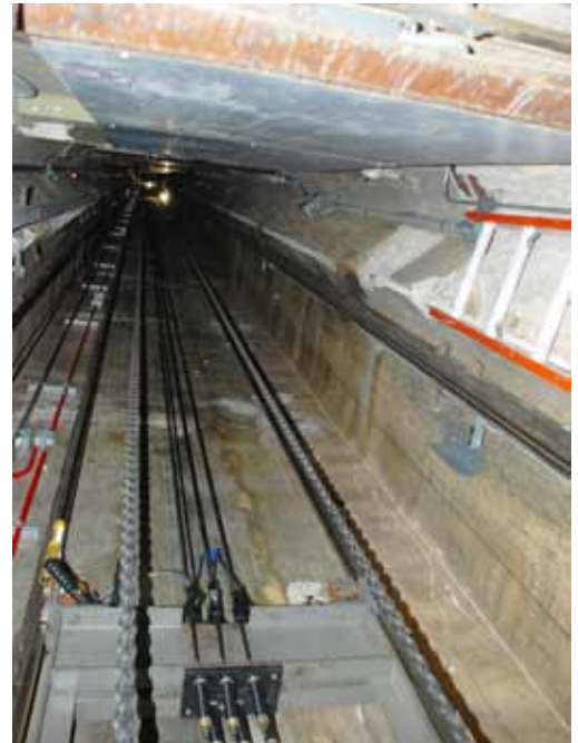
Looking into the elevator shaft at basement level reveals the new buffers, below, which would slow and stop the elevator in a fall. Above, the elevator shaft open to the 14th floor level.
