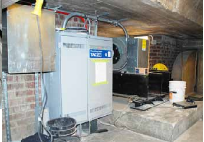
The 1980 era elevator equipment fills a machine room, left. New more efficient and compact elevator controls take up much less room, below.
