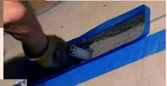
Once the non-original bar light was removed, OCC staff filled the slots cut into the limestone. It took a series of fills or lifts to bring the level back up to the surface of the stone. The final layer of mortar was color matched to the limestone.
