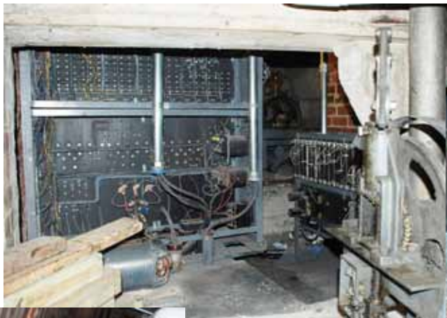
The 1980 era elevator equipment fills a machine room, left. New more efficient and compact elevator controls take up much less room, below.
