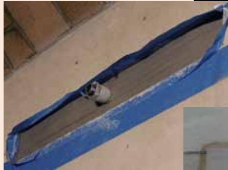
Once the non-original bar light was removed, OCC staff filled the slots cut into the limestone. It took a series of fills or lifts to bring the level back up to the surface of the stone. The final layer of mortar was color matched to the limestone.
