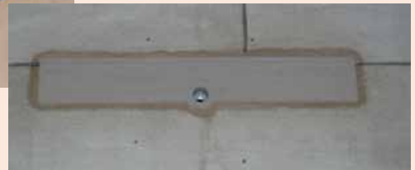
Once the non-original bar light was removed, OCC staff filled the slots cut into the limestone. It took a series of fills or lifts to bring the level back up to the surface of the stone. The final layer of mortar was color matched to the limestone.
