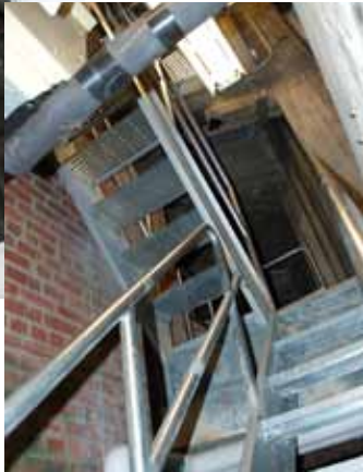
Access to 14th floor elevator equipment has been improved. The ladder above has been supplemented with stairs and a walkway, right.
