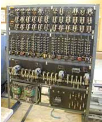
Above, a single computerized control panel has replaced two large mechanical switch panels, left, to control elevator movement.
