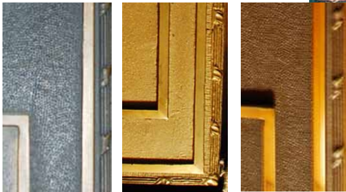
Finish details from, left to right, the original panel, the 1980's panel, and the new panel reveal the importance of having historic materials as examples.
