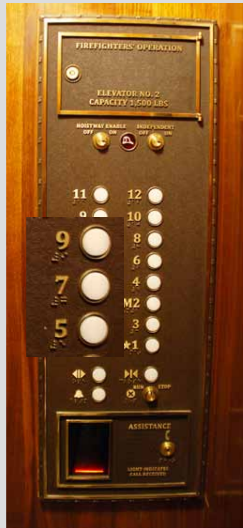
New elevator panel with braille added.
