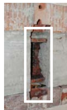
Steel beam uncovered, above. Slotted plate added for stability, below.
