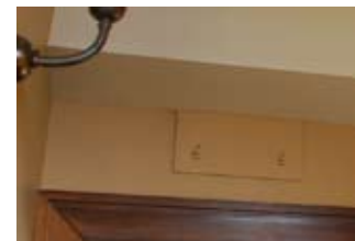
Steel beam uncovered, above. Slotted plate added for stability, below.
