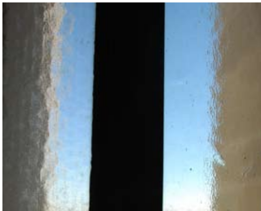
The vendor matched the color of the original glass, left, with only a slight variation in texture, right.
