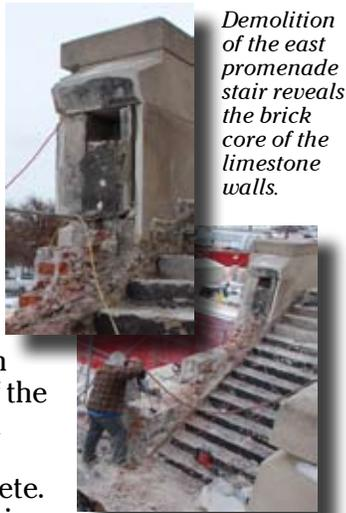
*Demolition of the east promenade stair reveals the brick core of the limestone walls.*
