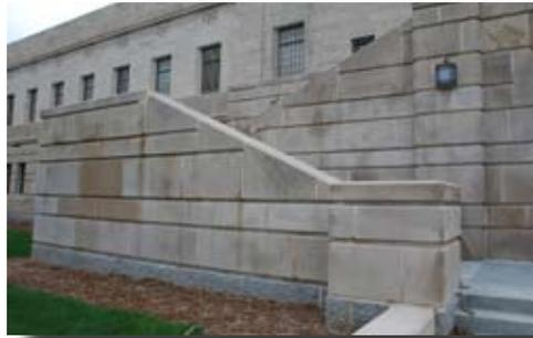
*The west promenade stair, newly restored, appears to be constructed of granite and limestone. The concrete and brick core are hidden from view.*
